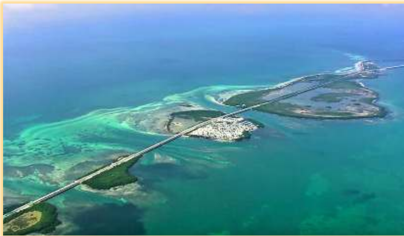
Image 12: An aerial view of the Overseas Highway, or U.S. 1, through the Florida Keys (Source: Florida Keys News Bureau)
