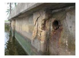
Figure 2.7.4 T-Pile Spall and Panel Cracking
