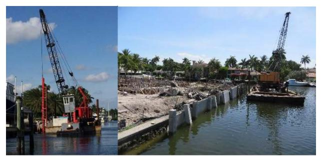
Figure 4.10.1 Conventional Seawall Installations
